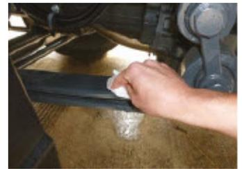
Loose paint and rust must be cleaned down to bare metal. The site must be dry before installation
