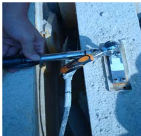
Fig.3 Load Link fitting
