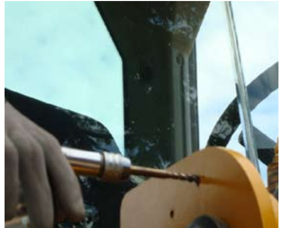
Fig.4 Tapping Weighing Zone bracket fixing points
